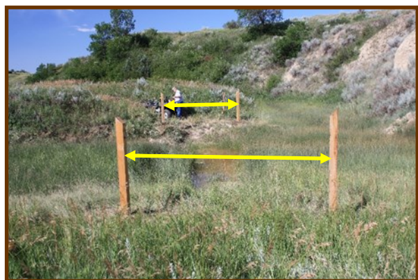
Buffalo Gap Trail submerged concrete slab Knutson Creek Crossing, July 19, 2018. Photo by Roger Ashley.
