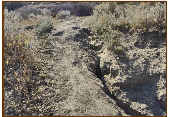
Erosion of a downslope section of trail
